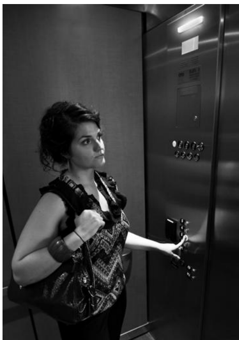
Emergency Lighting/Alarm Bell system provides passenger reassurance in emergencies
